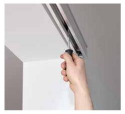
End stop and activator are easy to fit: Just screws on to the track. No pre-drilling necessary. No irritating aluminum chips in the profile. Positioning easily adjusted.
